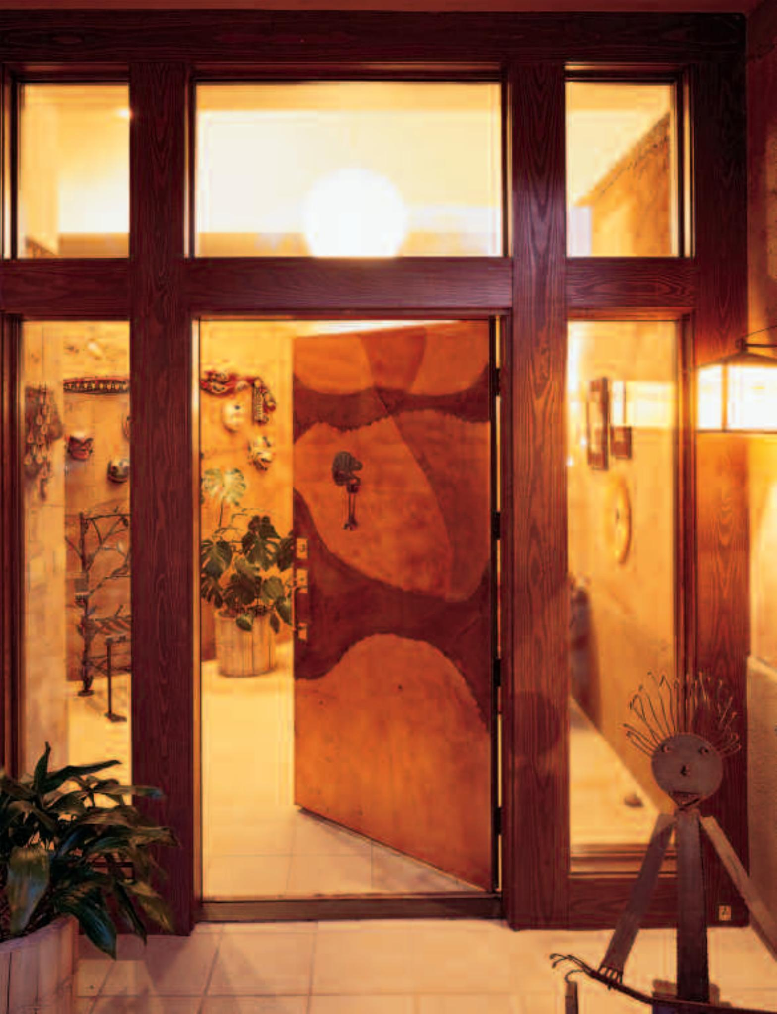
Frerking's wife, Joanne, a fabric and watercolor artist, consulted with Jan on color before adding pigments to the cast earth mix that resulted in the rich earth tones in these walls. The windows were set into openings in the cast earth walls and anchored with drywall covered with similarly pigmented earth plaster.
