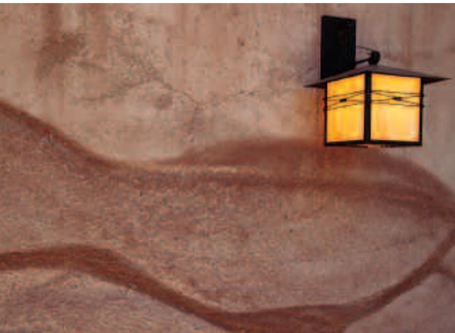
**ABOVE:** Contractor J. W. McShane etched a dark, wave-like pattern into the curved, exterior cast earth wall using a high-pressure hose. Jan went over the design with iron oxide and a wet sponge to add color.
